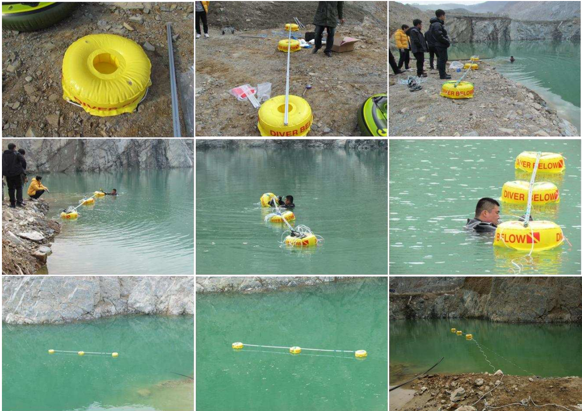
Figure 4.4 Installing buoys and aluminum profiles.
