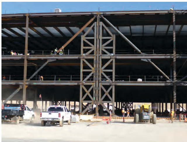
Fig. 8. (a) Elevation drawing and (b) photograph of strongback frame for the Tesla facility; (c) Krawinkler fuses (images courtesy of Gregory P. Luth & Associates).
